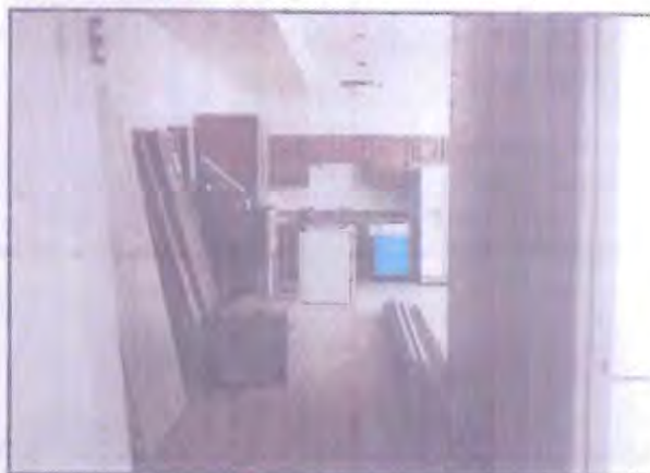
Appliances, doors and trim sit waiting to be installed into one of the new apartments that are being built from the old classrooms of the Hubbard High School.
