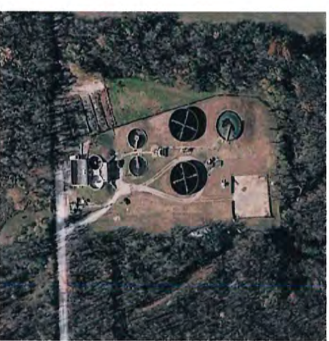
North WWTF (Pump Station)
