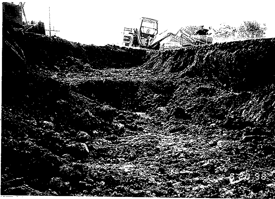
Main excavation. (Old Hudson Station, Sedalia, MO)
