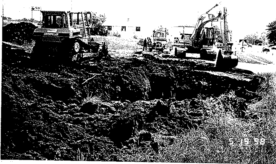
View looking east. Main excavation. (Old Hudson Station, Sedalia, MO)
