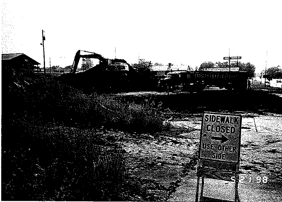
View looking east. Contaminated soil export. (Old Hudson Station, Sedalia, MO)
