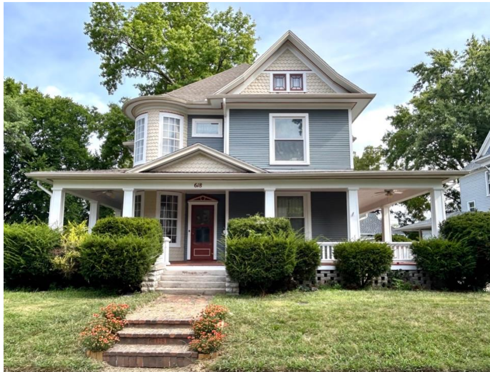
Photograph 3 Restoring Design Elements: Voluntary mitigation for this Queen Anne-Style home built c. 1910 might involve the replacement of the sash window located on east side (right) of the second story with a six-over-six multi-lite configuration. Location: 618 W. 6 th St., Sedalia, MO.
