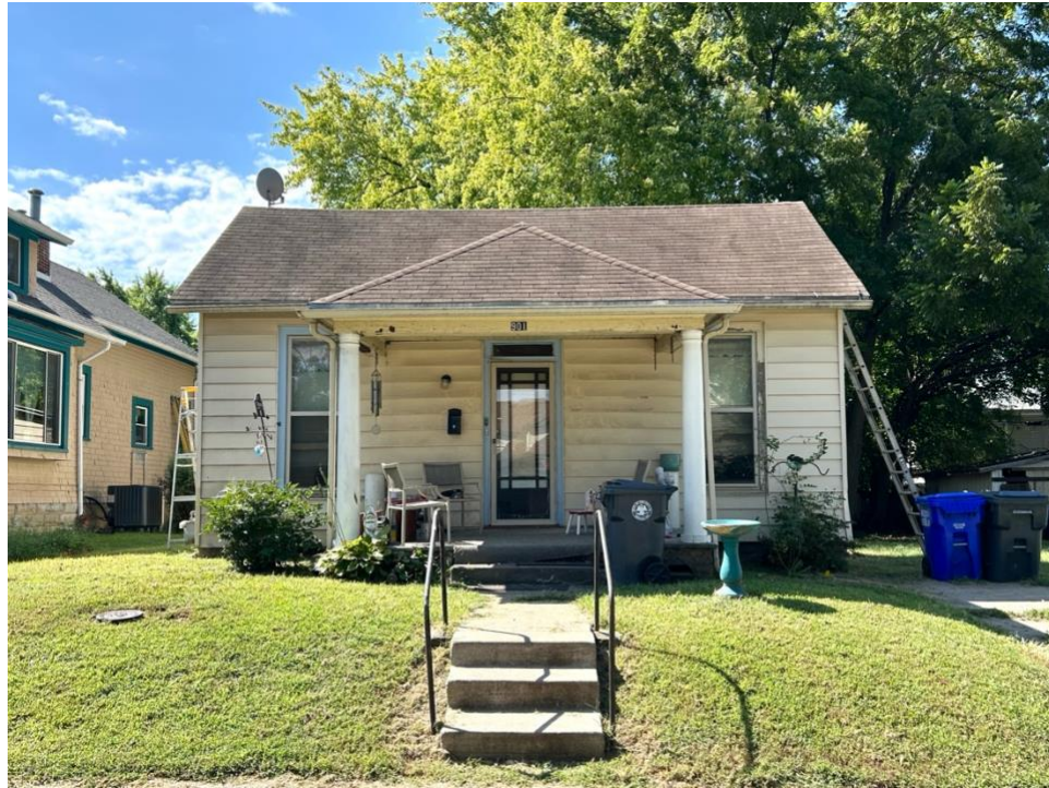
Photograph 14 Round Columns Decorate a Plain Folk Victorian-Style Dwelling Built c. 1880: This small house consists of a simple rectangular floor plan and a gabled roof. The porch has a hipped roof (SFS Architecture 2021:40). Location: 901 W. Fifth St., Sedalia, MO.
