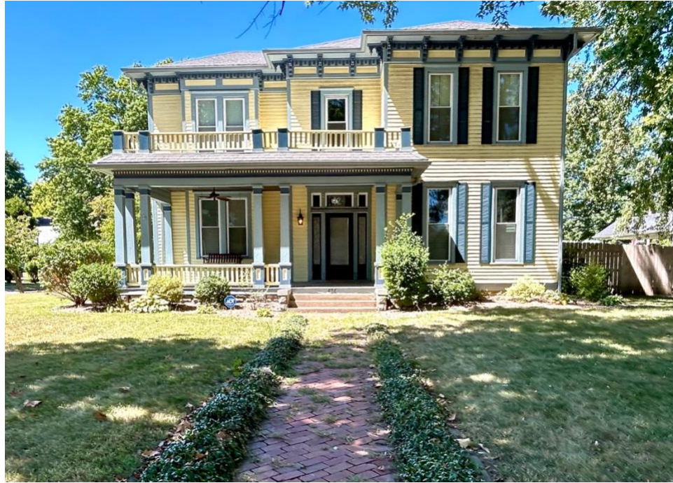
Photograph 11 Two-story Wood-framed Italianate-Style Dwelling Built c. 1890: The house features the original stone foundation, a hipped roof with bracketed eaves, and wood clapboard siding (SFS Architecture 2021:45). Location: 424 S. Grand Ave., Sedalia, MO.
