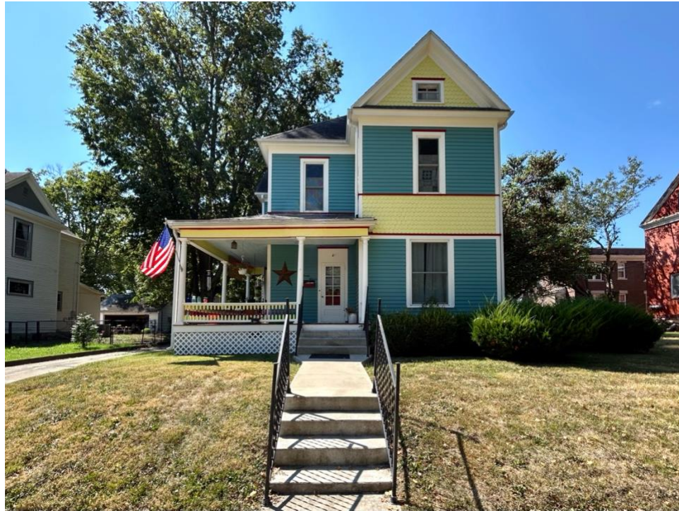
Photograph 12 Queen Ann-Style Dwelling Built c. 1880: This residence was once the home of James H. Barley of Farm Implements (Maserang 1985:86). The front and side gables of the L-plan are separated by a middle hipped section. Features include a wrap-around porch and fish-scale trim. Location: 711 W. Fifth St., Sedalia, MO.
