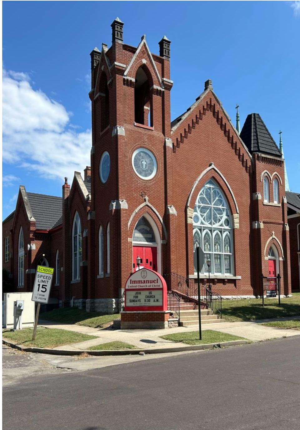
Photograph 16 German Immanuel Evangelical Church Built c. 1896: This Gothic Revival-Style building demonstrates the influences of German craftsman in the steep hipped roof over the east tower, decorative brick work along the roof, stepped roof shingles, and the four intricate finials on the square west bell tower. The brickwork with sandstone detailing and stained glass windows are examples of the traditional aesthetic that immigrants contributed to the City of Sedalia. At the time that this church was built, at least twenty percent of the local residents were first generation German immigrants (SFS Architecture 2021:43). Location: 418 W. Fourth St., Sedalia, MO.
