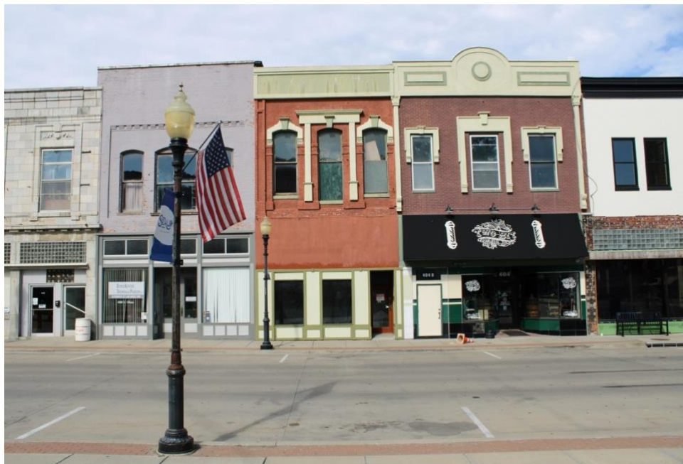
Photograph 8 Vernacular Commercial-Style Storefront Built c. 1883: This brick storefront was covered with aluminum and architectural glass in the 1940s. The second story has aluminum panels and gold aluminum sheathing. This resource is rated as non-contributing to the Sedalia Commercial Historic District (NRHP NO.: 01000687), but it is an excellent example of a 1940s storefront (Alice Edwards 1993:12). Location: 406 S. Ohio Ave., Sedalia, MO.
