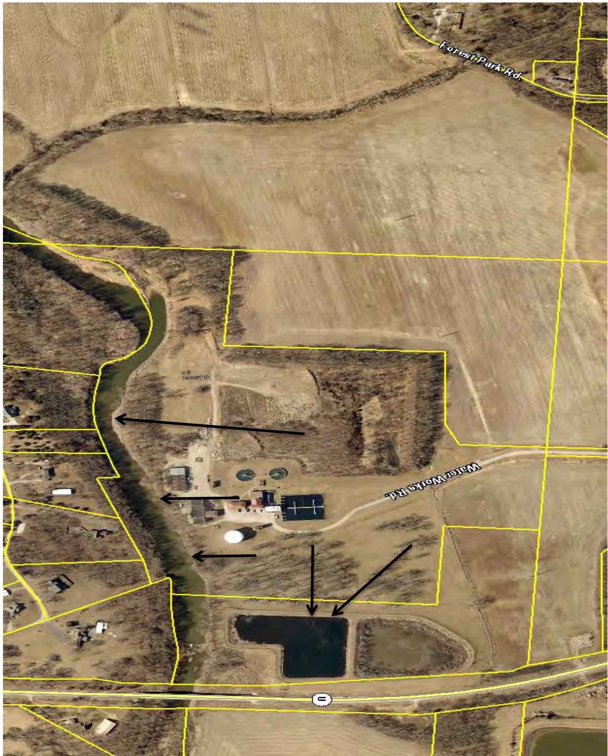
Figure A-18 Water Treatment Plant / Water Division – Water Drainage
