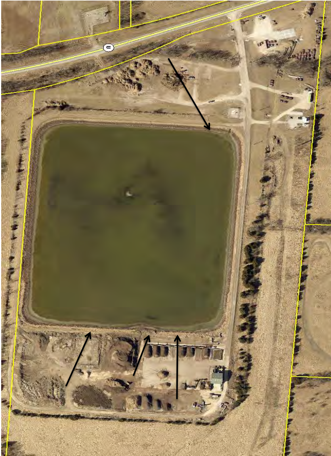
Figure A-22 Compost Facility – Water Drainage
