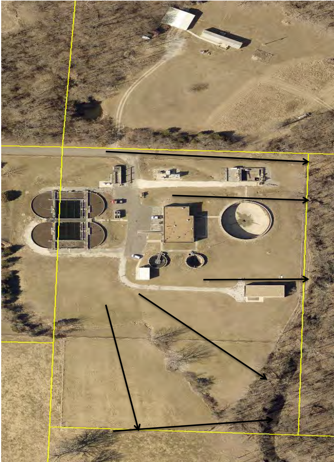
Figure A-21 Southeast Wastewater Treatment Plant – Water Drainage
