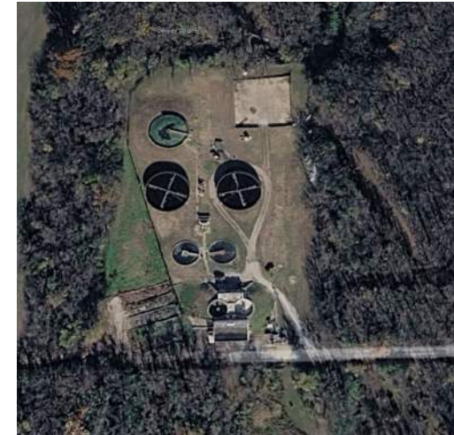
North WWTF (Pump Station)
