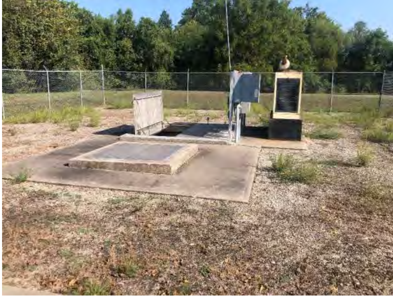
Figure 2 32 nd Street Lift Station
