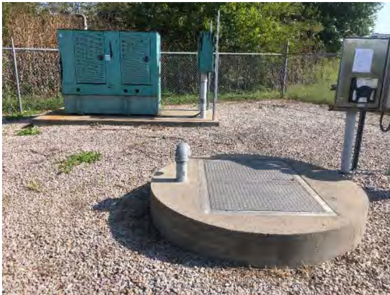
Figure 1 16 th Street Lift Station
